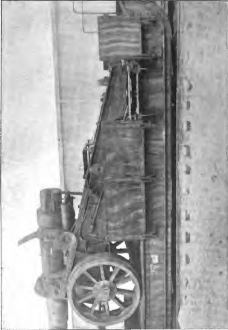
CARRIAGE FOR THE 170 MM. GERMAN GUN (RECOIL AND ELEVATING MECHANISM).
